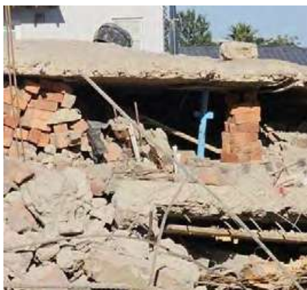
Consulting engineer placed on precautionary suspension following building collapse
